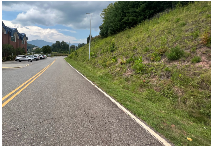
Image 8. Steep Grade along Cliffside Drive
