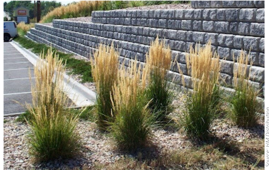
Image 36. Retaining Wall Example
