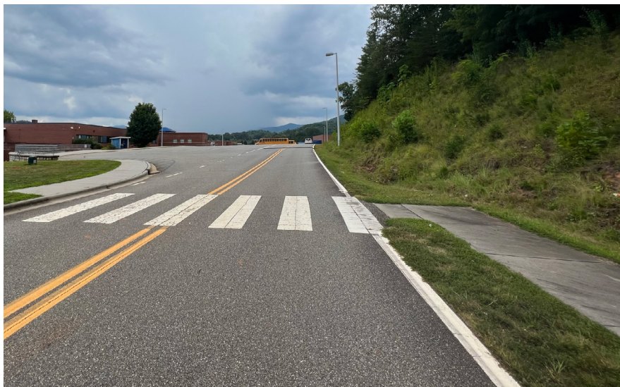
Image 10. Crosswalk on Cliffside Drive
